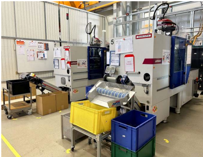
Fig. 2: 15 injection molding machines are installed at the plant, ready to produce a great variety of different plugs and connectors. The newest machines are two SmartPower models from WITTMANN. The WITTMANN machines' energy efficiency was the decisive argument in the decision-maker's choice.
