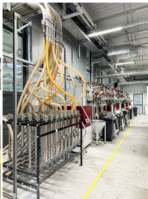
Fig. 4a+b: The granulate is fed into the materials handling system with gram-accurate precision by Gravimax gravimetric blenders from WITTMANN.
